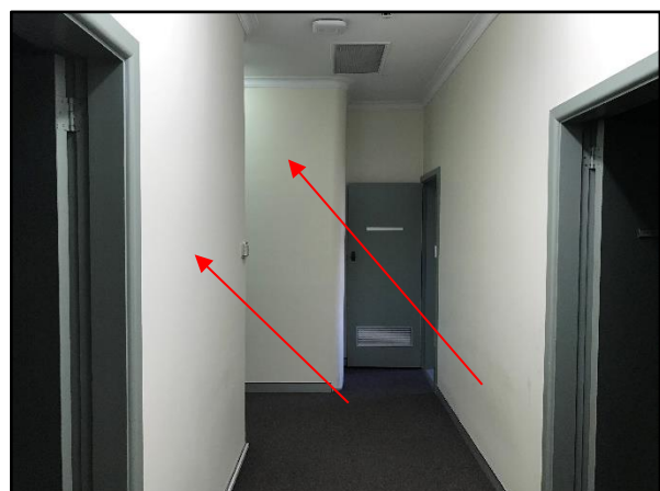
Figure 17. View to the internal corridor. The red arrows indicate the curved masonry walls.
